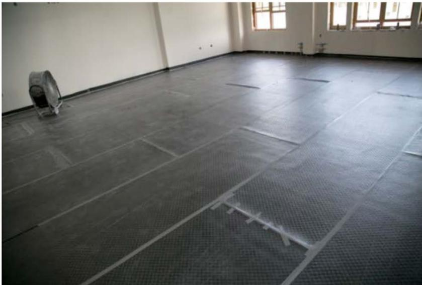
7. Use **GenieMat<sup>®</sup> PMI** to wrap all columns, drains, penetrations to ensure there is no hard surface contact with the topping material (plywood or concrete).
